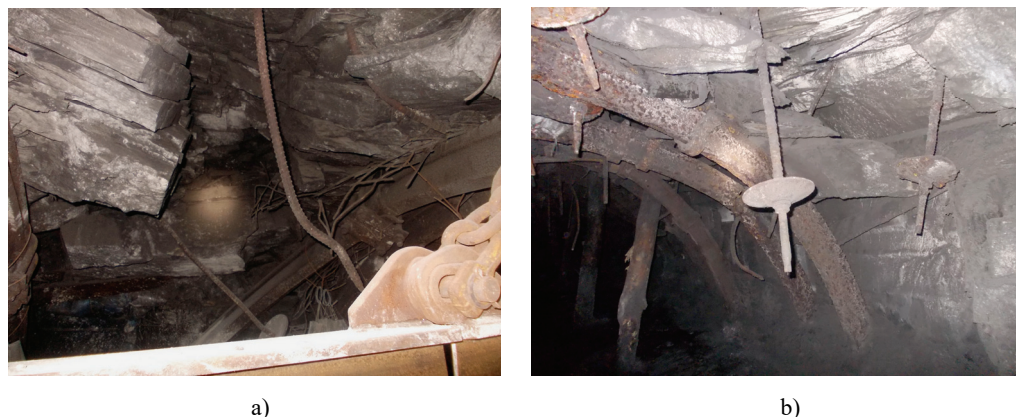
Fig. 1. Rock falls in mine roadway supported by rock bolts: (a, b) Management Board of the “Pokrowskoje” mine, Ukraine (authors’ photos)
