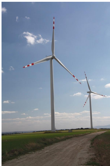
Fig. 2. Part of the Lipniki wind farm in the Kamiennik commune ( Nyski powiat) (source: http://www.tauron-ekoenergia.pl/elektrownie/energia-z-wiatru/farma-wiatrowa-lipniki )
